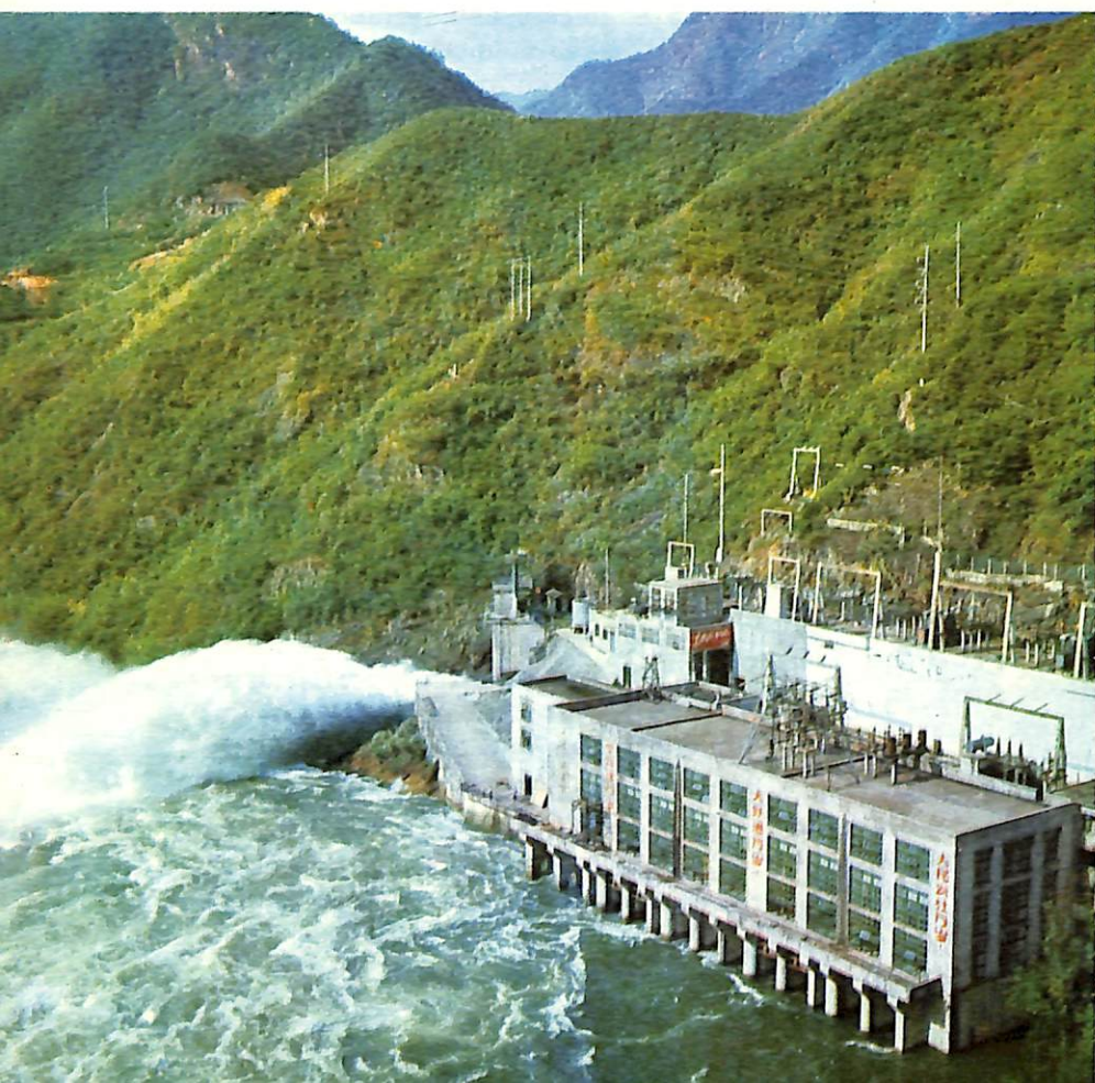
A hydroelectric power station on a large reservoir.
